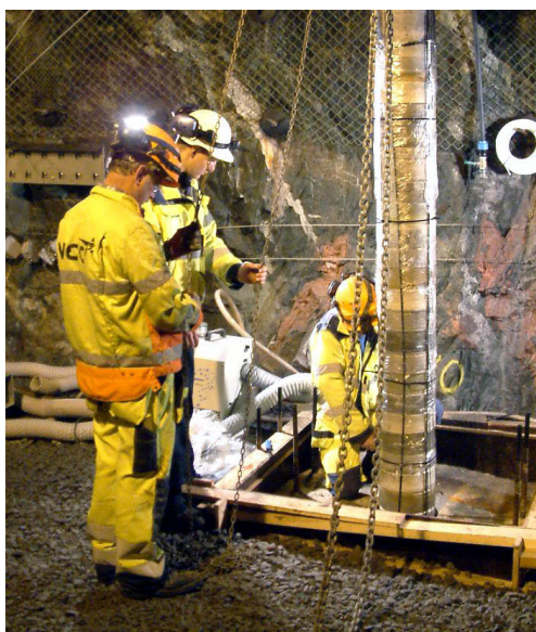
Installation of one of the three packages illustrating the mixing of the different compacted buffer discs.
