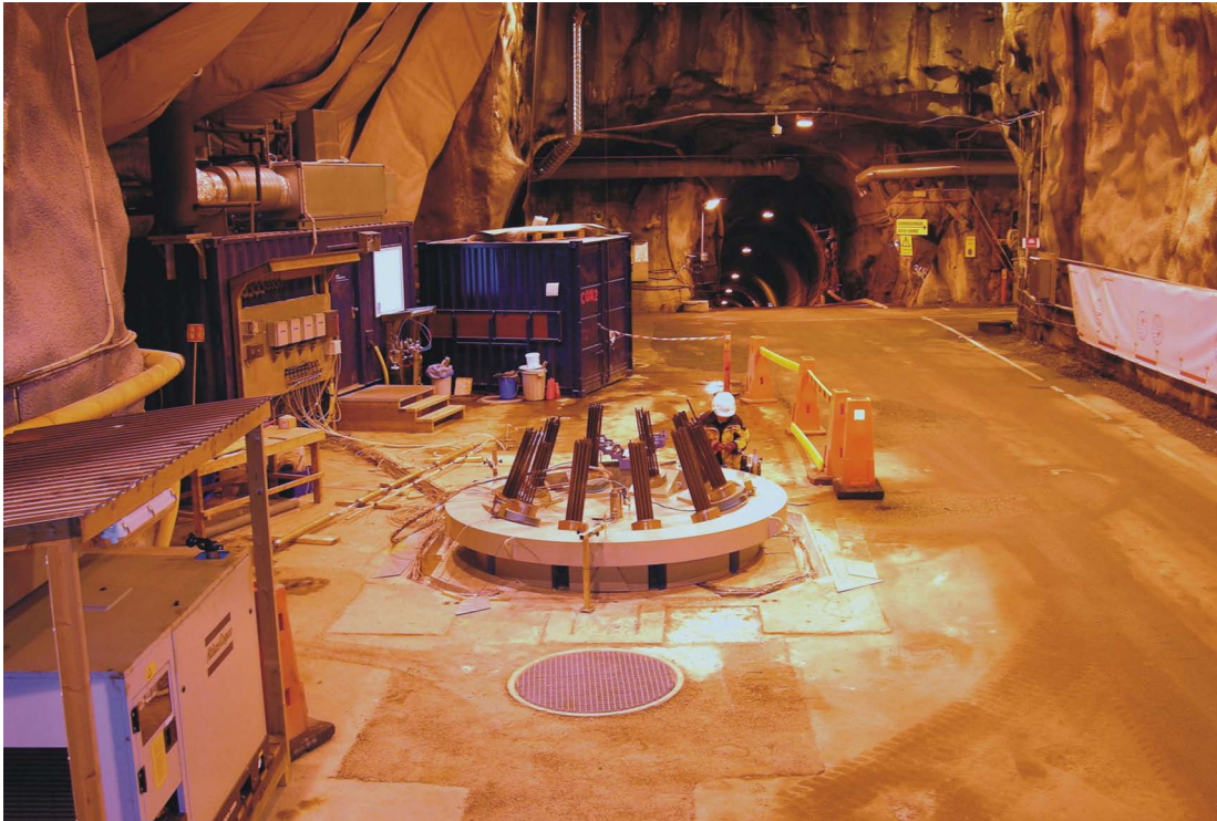
Large-scale gas injection test (Lasgit) 420 m below ground at Äspö HRL. A scientist from the British Geological Survey (BGS) works next to the large steel lid anchored over the deposition hole.
